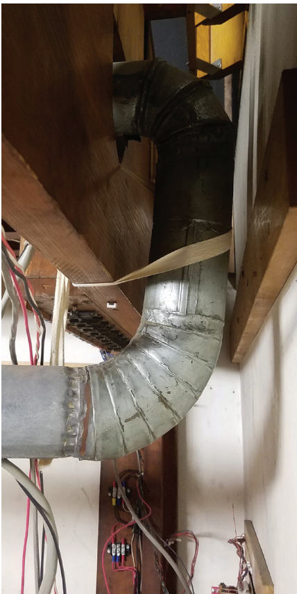
9. (left) This windline is being held in place by a rope, and it still leaks a lot of wind.
